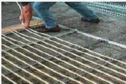
Manufacturing the pipe grid
