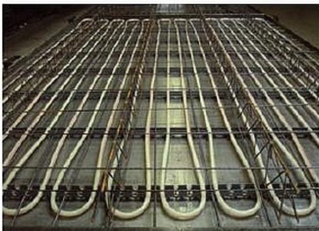
Prepared pallets with pipe grid and reinforcement
